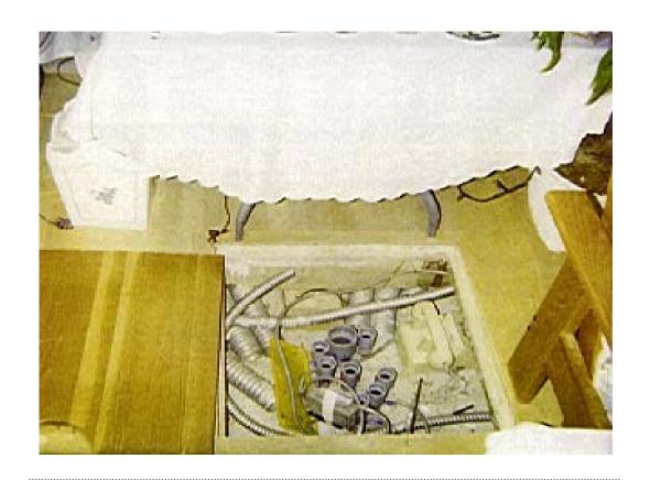
Uncovered electrical conduit: one pipe had a 2" diameter and the others a 1" diameter
